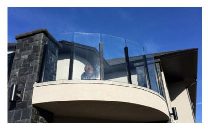
Panorama Universal Post allows a 30 degree angle in both directions for a full 60 degree variance for custom deck designs. Curved decks are easily accommodated with Panorama Universal Post.
