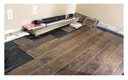
Laminate flooring, a popular material. It is available at affordable price; it is easy to install and its durability is outstanding. This surface is compose of an inner core of either fiberboard, or resin material, combined with a photo application layer through a lamination process. Laminates are an intriguing affordable alternative to hardwood, ceramics, and stone tile, not the most affordable material. Laminates surfaces are ideal for active families. Beware of its vulnerabity to moisture.
