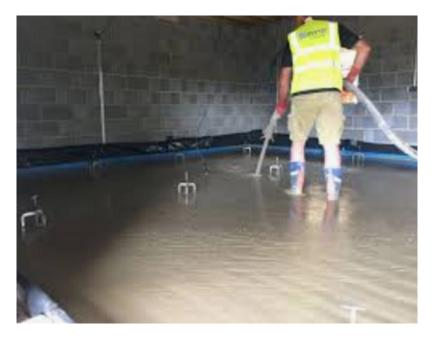
Rapidly pumped into small or large areas, it really is a cost-effective alternative to concrete and other flooring solutions. The chemical composition is actually quite similar to ready-mix concrete, however with fewer and finer aggregates.
