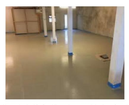
This quick-drying liquid screed, valued for flowability, makes a smooth interior surface with underfloor heating systems. This flush coating for heating pipes is virtually void-free and bubble-free. With significantly lower drying times compared to calcium sulphate liquid screeds, it allows the floors to be used in half the time typically required for the gypsum screeds in residential, commercial, and large-area industrial environments.
