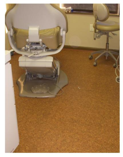
It is an interlocking flooring product customized for use in hospitals, cleanrooms and labs. It's water-proof seam sealer makes tiles liquid-tight but still removable and replaceable. It is a useful feature for those labs and clinics using chemicals that if they are inadvertently spilled and if it is allowed to seep into flooring underneath may be damaging and dangerous.
