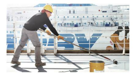
Also, the continuous waterproof membrane can be used as a levelling compound. Sika has many designs and colors, which provides designers with the freedom to design logos and cutting planes. Combine the colors, which were tested for over 5,000 hours: encouraging stability.
