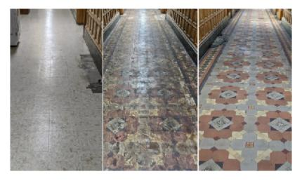
These vinyl squares, installed decades ago, were covering <u>encaustic tile</u> with a geometric pattern original to the building. The tile was under asbestos. Initially, it didn't seem salvageable? But, after a thorough remediation and cleaning process, the English encaustic tiles installed at the turn of the 20th century looked impressive. It was an amazing transformation.
