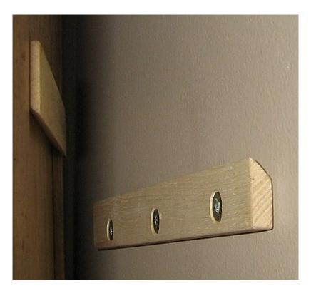
No. It has nothing to do with footwear or sports. It is something else, entirely. A French cleat is actually a <u>molding</u> with a slope angled at 30 to 45 degrees. It is a weight bearing molding effective for mounting a heavy object to a wall.
