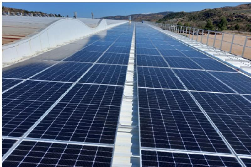
[Photovoltaic](#) panels with a system size of 1,212 kWp have been installed are capable of meeting 25% of the company's annual demand for electricity; through its manufacturing plants. Estimated yearly capacity's about 1870 MWh of electricity, which translates into an annual reduction of 374 tonnes of CO2 emissions; a substantial contribution to the decarbonization of its activities. These farms cover a combined 3,000 square meters on rooftops
